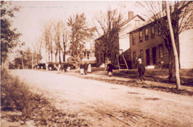
Above: Mill housing along Burden Lake Road
